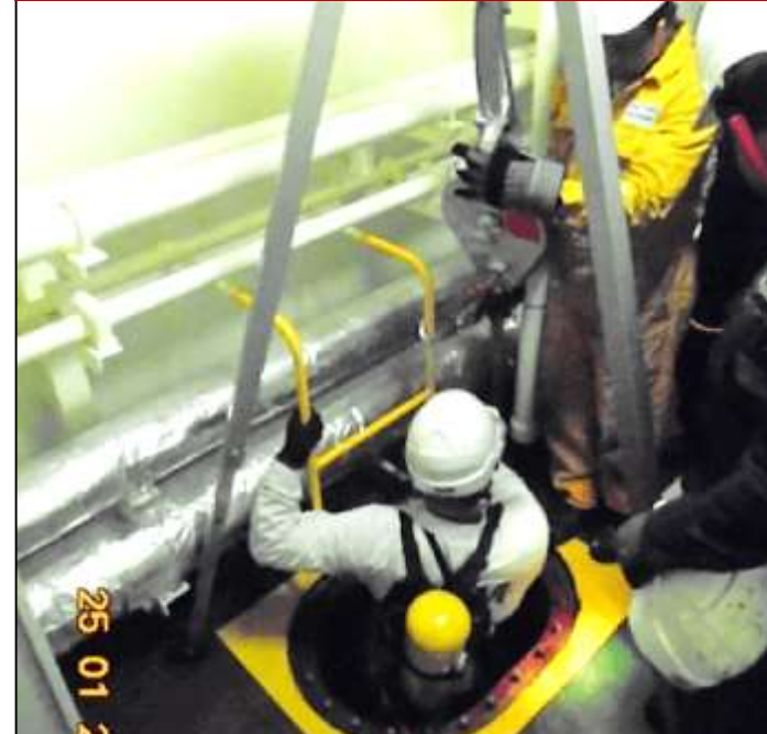
Hoisting/ Rescue/ Evacuate
